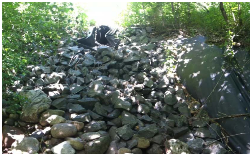
Figure 26. Representative Photographs of the Outlet Instability at 25524 Goodwin Road
