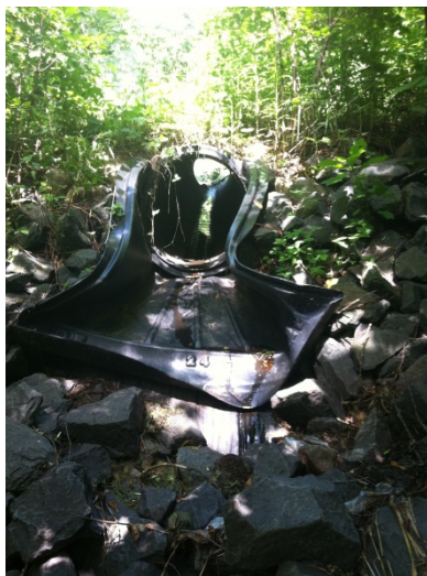
Figure 26. Representative Photographs of the Outlet Instability at 25524 Goodwin Road
