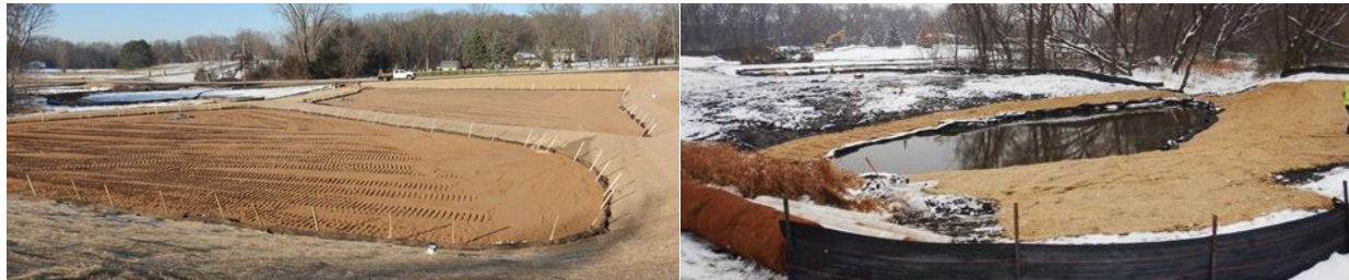
Project Construction: (Left) Iron Sand Filter Beds, (Right) Ditch Intake Pool
