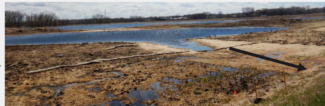
Location of the outflow of the pipe under Hwy 61 .
