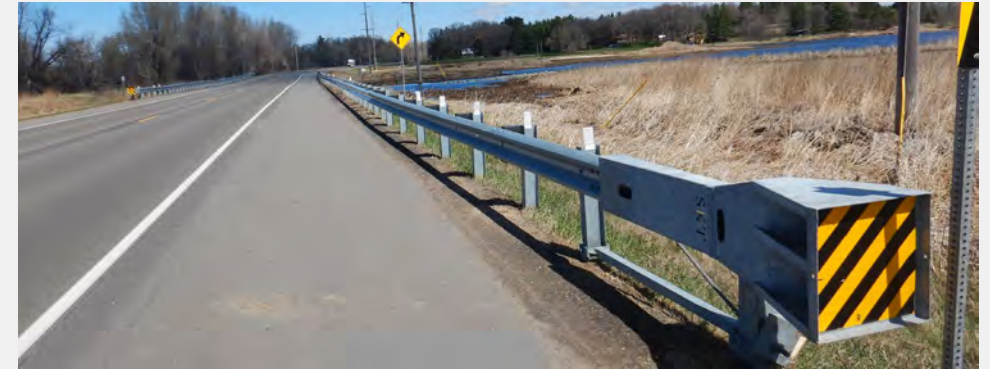
Guardrail extension installed 04-21-23
