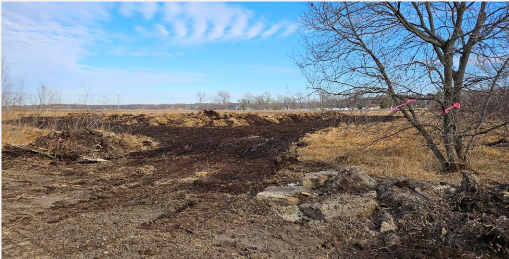
Early site prep in December.
