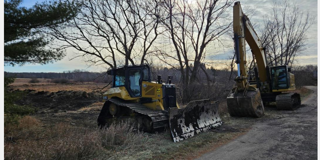
Equipment staged on site.
