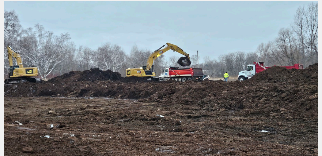
Excavation and haul.
