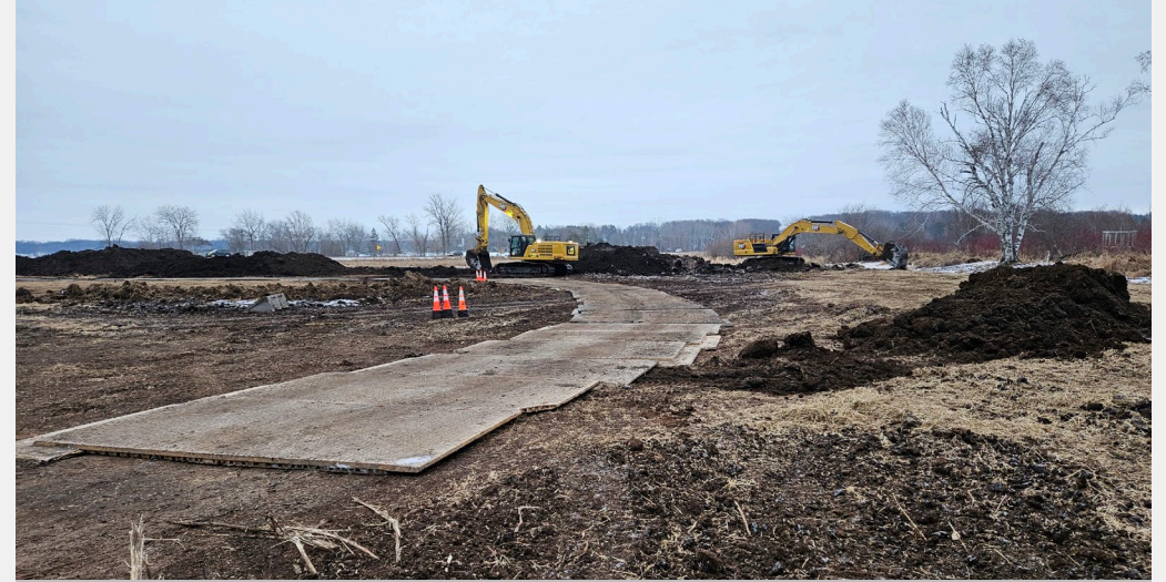
Matted haul road needed due to warm conditions.
