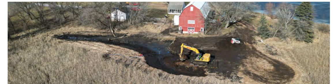
Photo: Moody Lake Capstone wetland dredging in-progress
