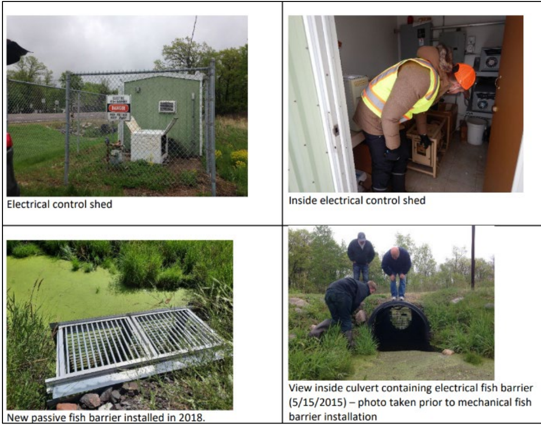
Figure 9 - Images of Electrical and Physical Fish Barriers between Shields and Forest Lakes
