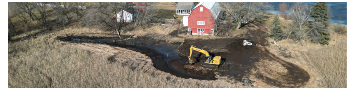
Photo: Moody Lake Capstone wetland dredging in-progress
