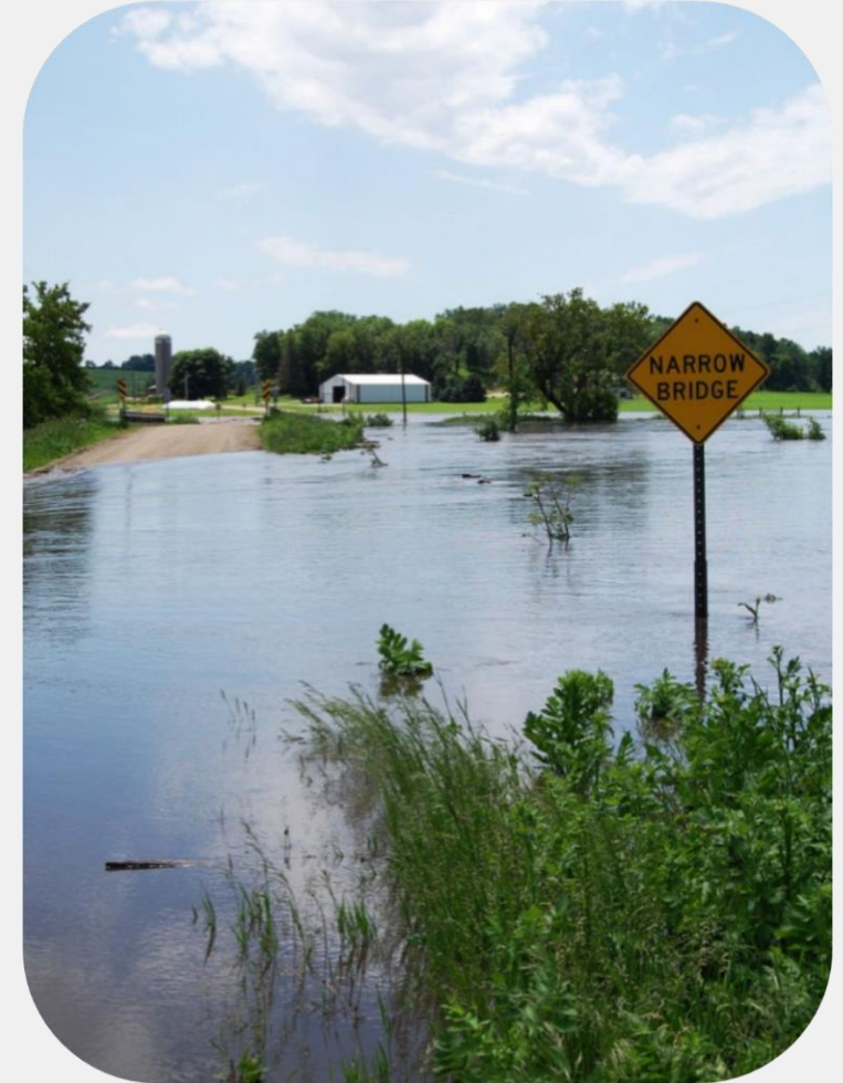
Example of Flood Risk – Road Flooding
