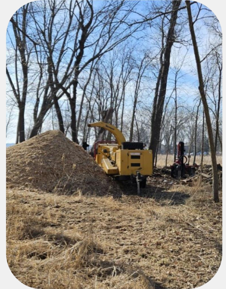
North Shore Trail Nature Area Hazard Tree Removal and Cleanup
