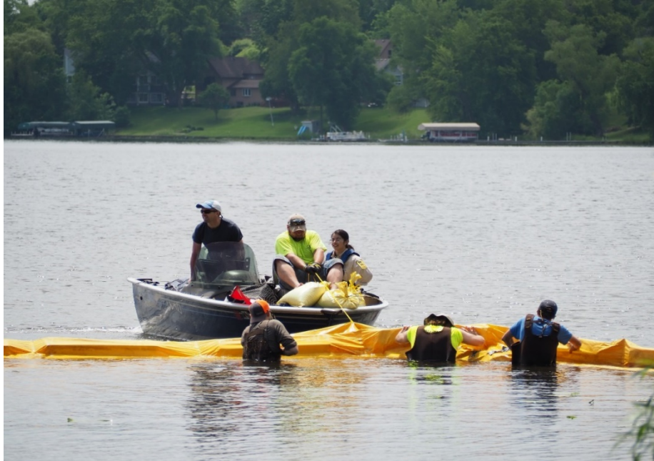
Figure 5 – Pulling the Barrier’s Corner into Position
