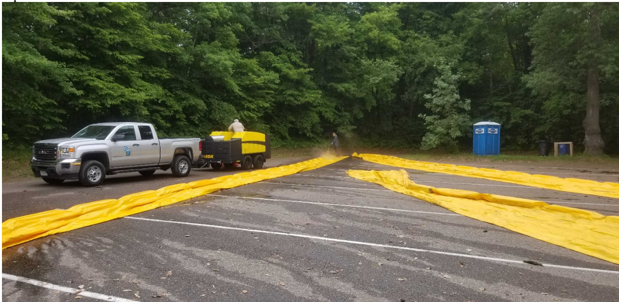
Figure 7 – Decontaminating Barriers after Removal
