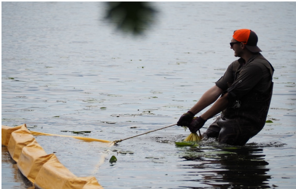
Figure 6 – Weighting the Barrier with Sandbags
