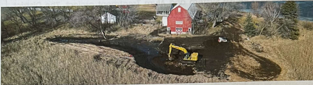
Photo: Moody Lake Capstone wetland dredging in-progress
