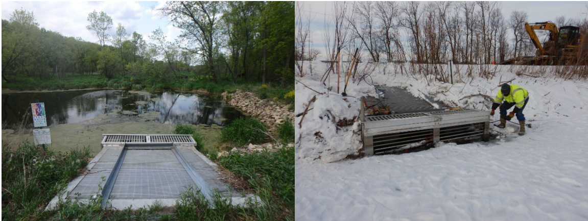
Figure 8 - Photos of Bone Lake Fish Barriers (Left Photo: Bone Lake Inlet Barrier. Right Photo: Bone Lake Outlet Barrier)
